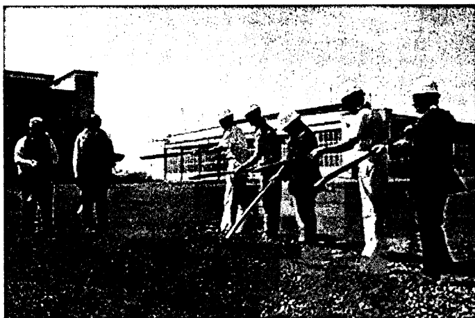
Senator Inouye, third from right, participates in the groundbreaking and blessing of NOAA's new Pacific Regional Facility on Ford Island.
