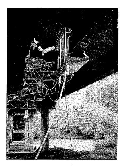
Figure 7. The end-effector in action under the bridge deck.
