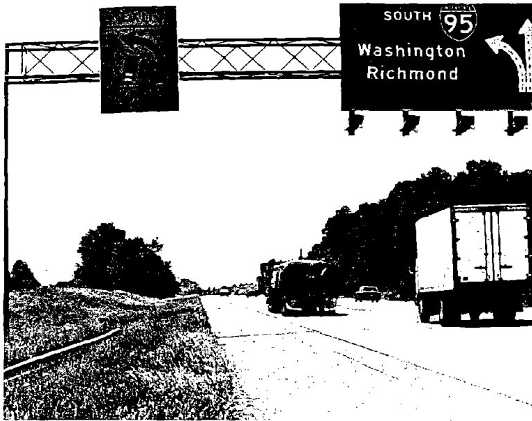
Figure 6. Sign being tested on the Washington, DC, beltway.
