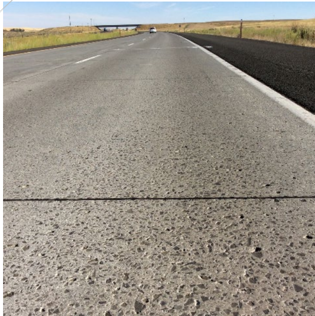
Figure 30. Section 530212, 900 psi, 11” PCC, 4” PATB, 4” DGAB. August 2017. Tining visible, no cracks or spalls.
