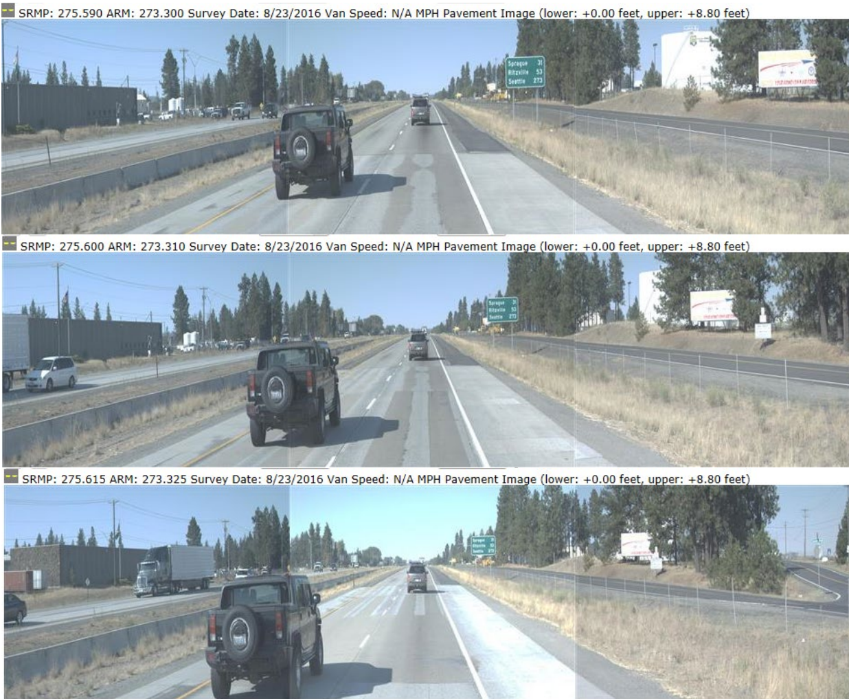
Figure 12. 2016 WSPMS views of the three polyester concrete sections. Top photo is of the screeled to fill existing ruts, middle photo is the grind and inlay the wheel paths, and bottom photo is the grind and inlay entire lane.
