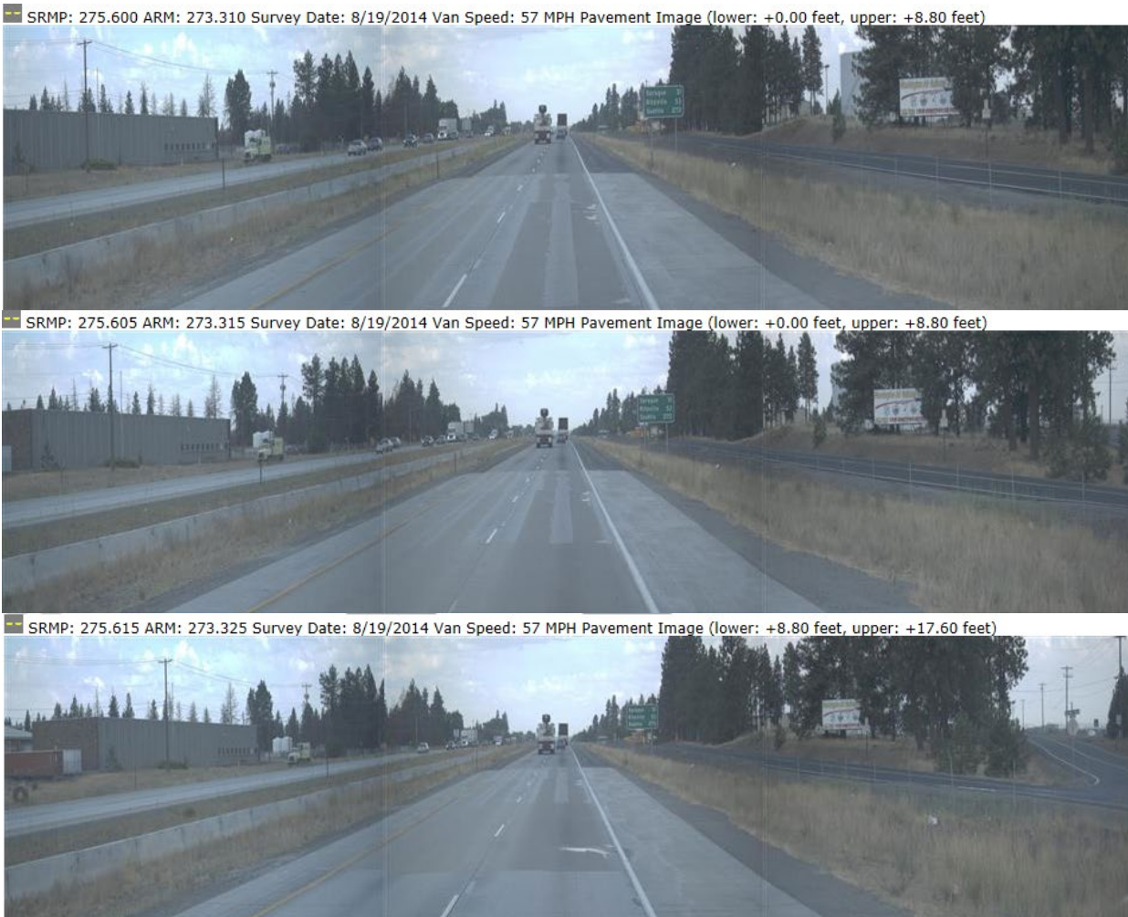
Figure 11. 2014 WSPMS views of the three polyester concrete sections. Top photo is of the screed to fill existing ruts, middle photo is the grind and inlay the wheel paths, and bottom photo is the grind and inlay entire lane.
