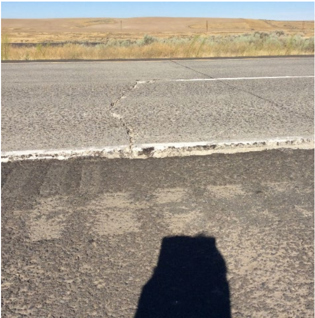
Figure 33. Section 530205, 550 psi, 8" PCC, 6" LCB. August 2017. No tining visible, three transverse cracks with spalling.
