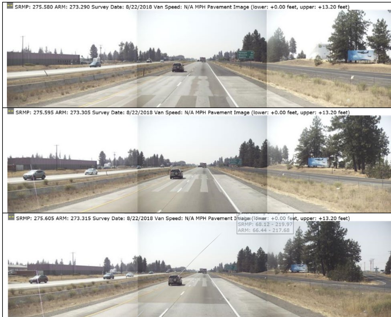
Figure 13. 2018 WSPMS views of the three polyester concrete sections. Top photo is of the screed to fill existing ruts, middle photo is the grind and inlay the wheel paths, and bottom photo is the grind and inlay entire lane.
