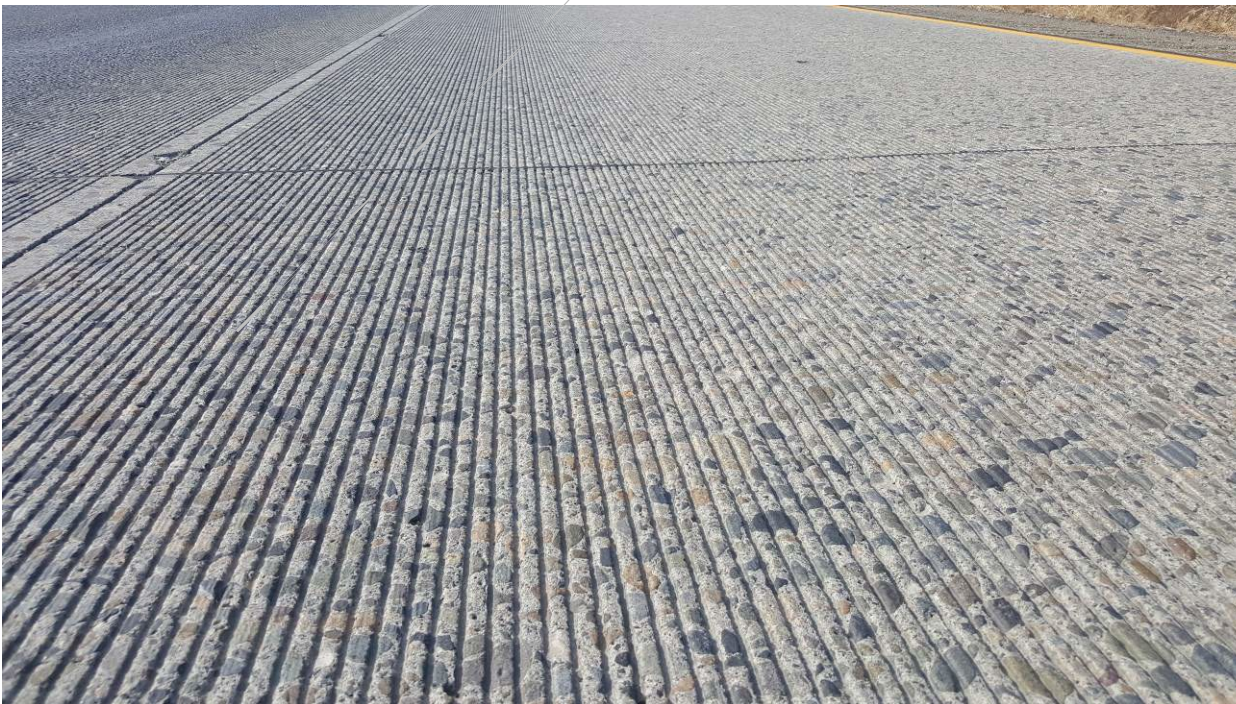
Figure 5. Note erosion of the edges of the land areas on the NGCS. October 2017.
