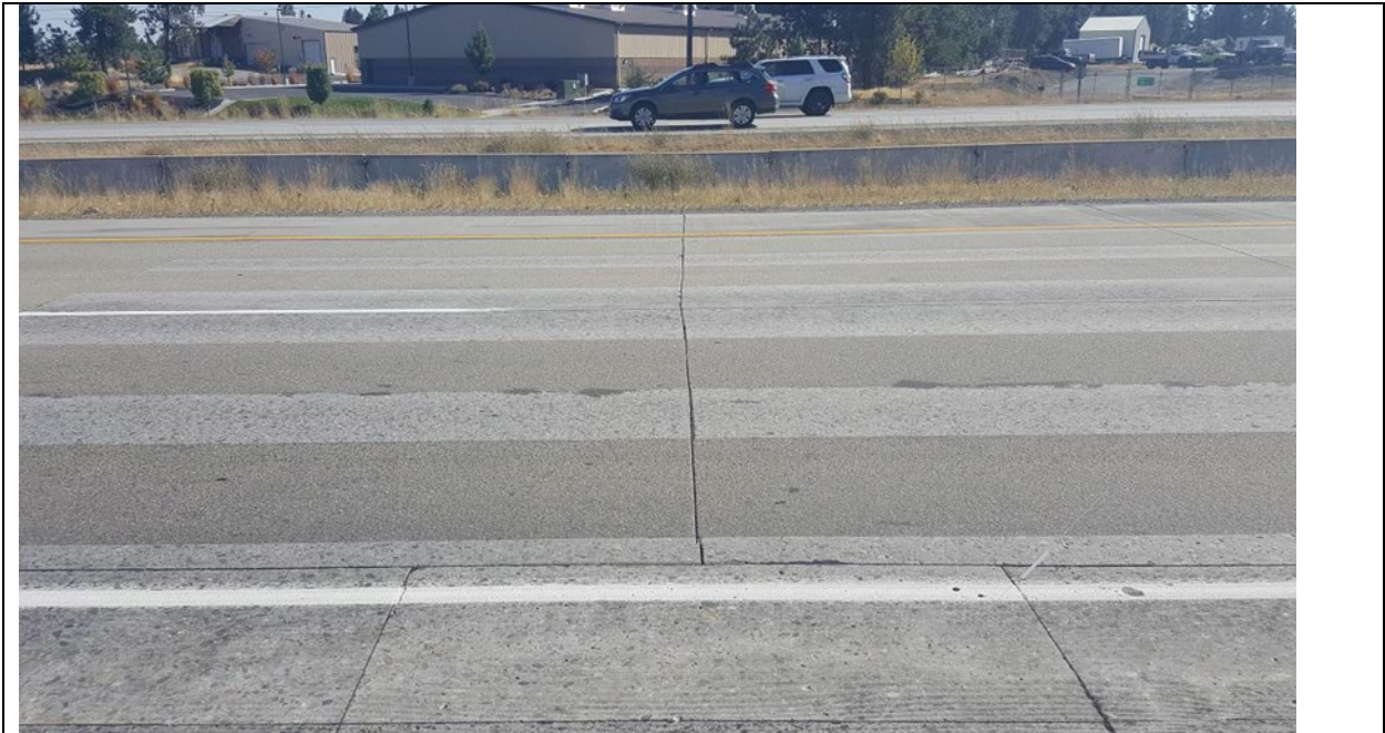
Figure 16. The wheel path one inch inlay section of polyester concrete. (Sept. 2017)
