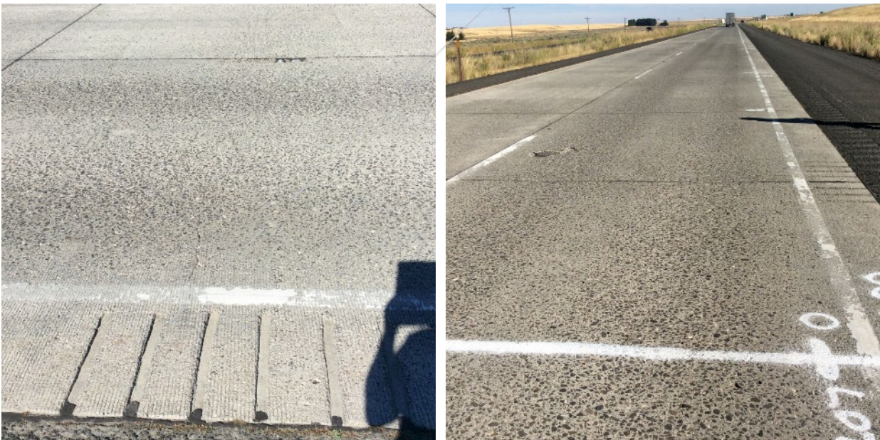
Figure 39. Section 530207, 550 psi, 11" PCC, 6" LCB. August 2017. No visible tining, three HMA filled potholes in the left wheel path. See Table 11 for summary of condition information for each section.
