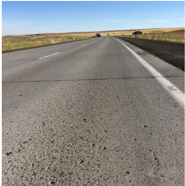
Figure 26. Section 530210, 900 psi, 8” PCC, 4” PATB, 4” DGAB. August 2017. Some tining visible, no cracks.
