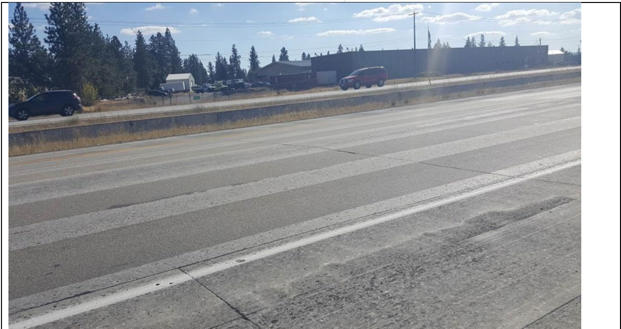
Figure 17. The wheel path one inch inlay section. (September 2017)
