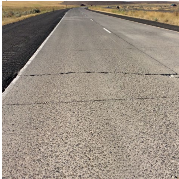
Figure 33. Section 530205, 550 psi, 8" PCC, 6" LCB. August 2017. No tining visible, three transverse cracks with spalling.
