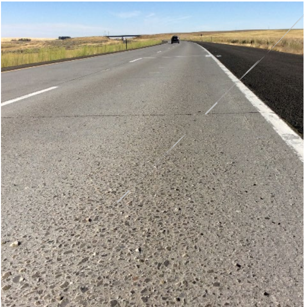
Figure 29. Section 530212, 900 psi, 11” PCC, 4” PATB, 4” DGAB. August 2017. Tining visible, no cracks or spalls.
