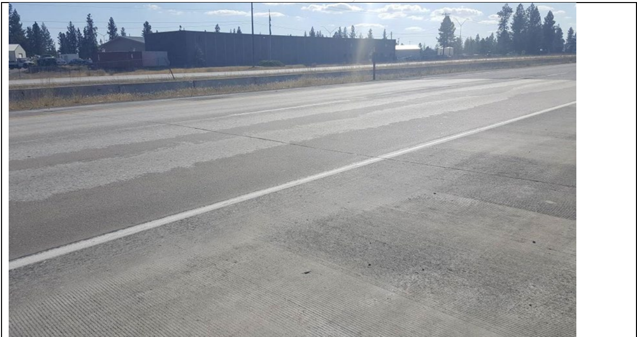
Figure 19. The screed to fill section of polyester concrete. (September 2017)
