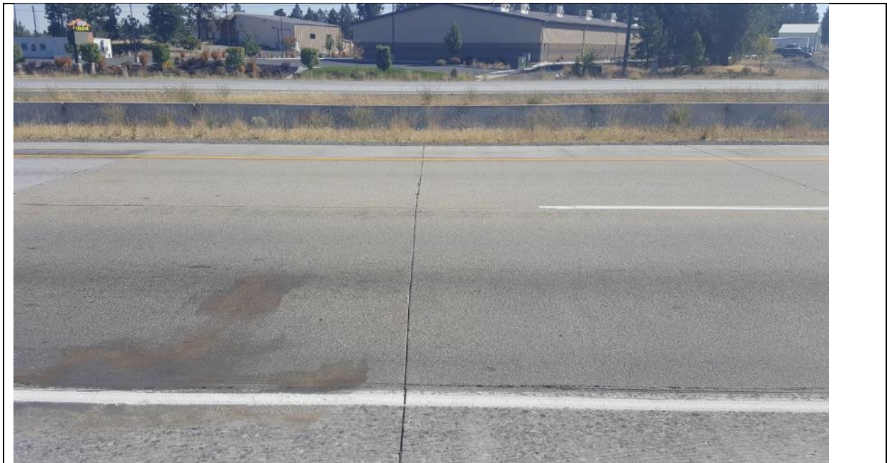
Figure 15. The total lane, one inch inlay section of polyester concrete. (Sept. 2017)
