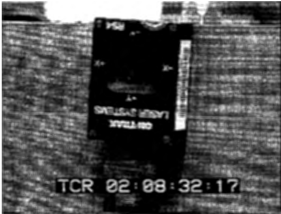
Figure 30. A laser receiver used to align the pipe section in the trench.
