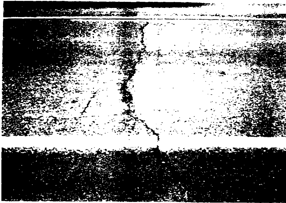
Figure 1. Typical Transverse Crack.
