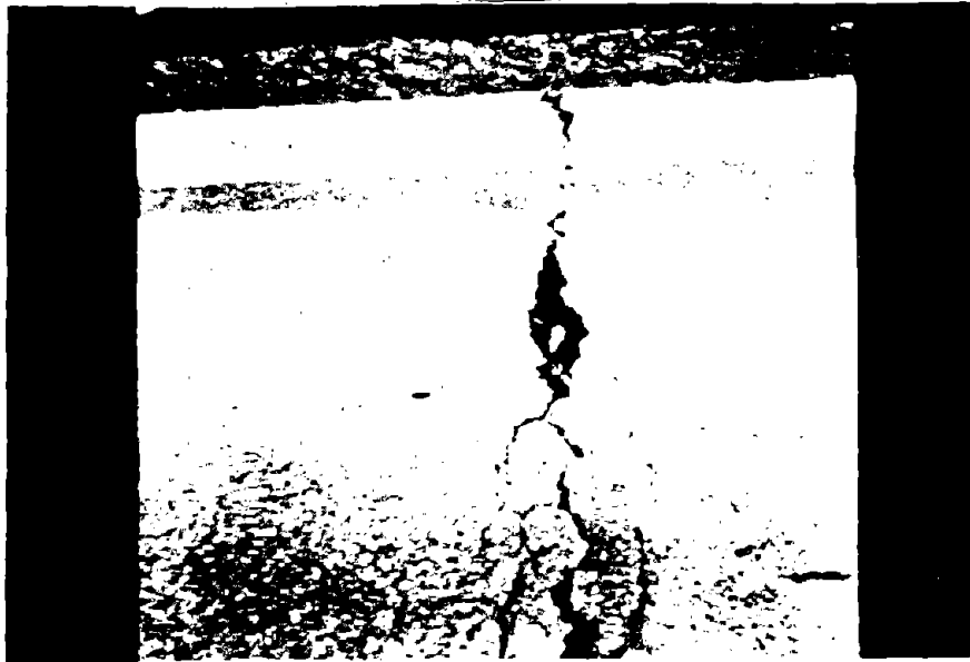
Figure 14. Joint Deterioration Due to Moisture.
