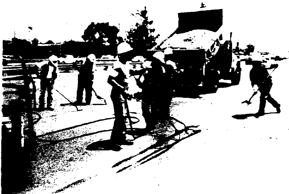
Figure 9. Longitudinal and Transverse Crack Filling.
