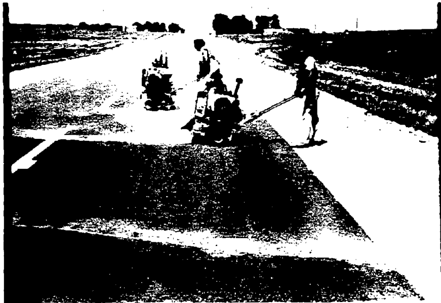
Figure 5. Routing of Transverse Cracks.
