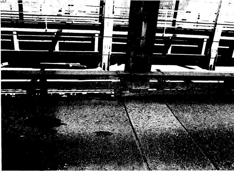
Figure 27. View showing roadway joints and discontinuous splash plates along edge of Williamsburg Bridge Roadway.
