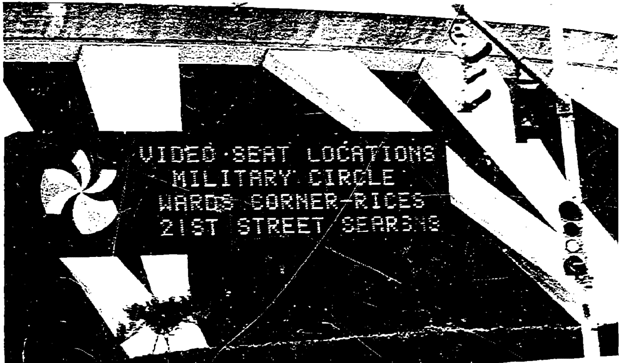
Figure 13. Burned-Out Lamps on a Message Center Sign Utilizing Sequential Display. (Source: Virginia Highway Research Council)
