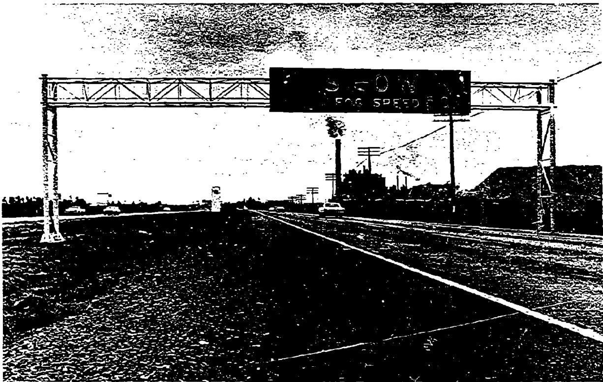
Figure 4B. Neon Sign Installation on I-5 Near Albany, Oregon. (Source: Oregon Department of Transportation)
