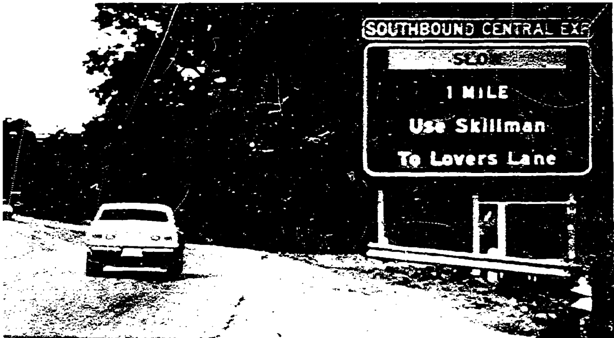
Figure 3B. Rotating Drum Sign Installation in Dallas, Texas. (Source: Dorsey, 1977)
