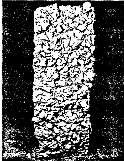
Underside of 3-ft by 1-ft by 6-in. slab bonded to saturated water-bound macadam base after test.
