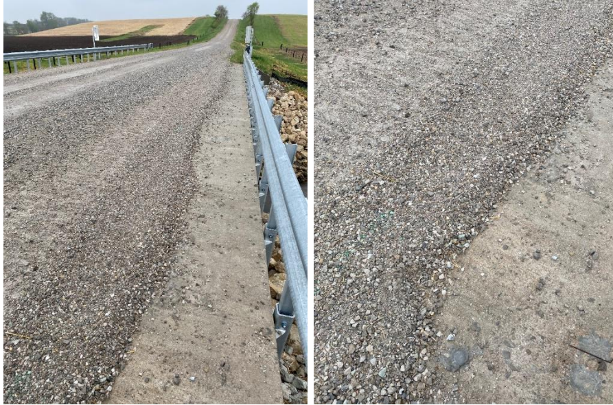
Figure 36. Top surface of the bridge deck – May 2021
