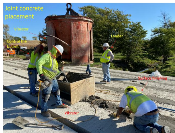
(d) Work crew during concrete placement
