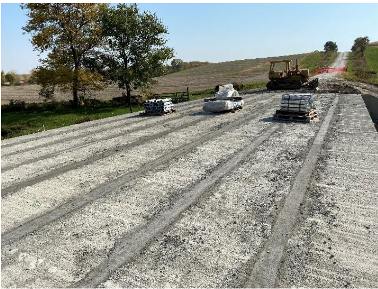
(a) Bridge top surface
