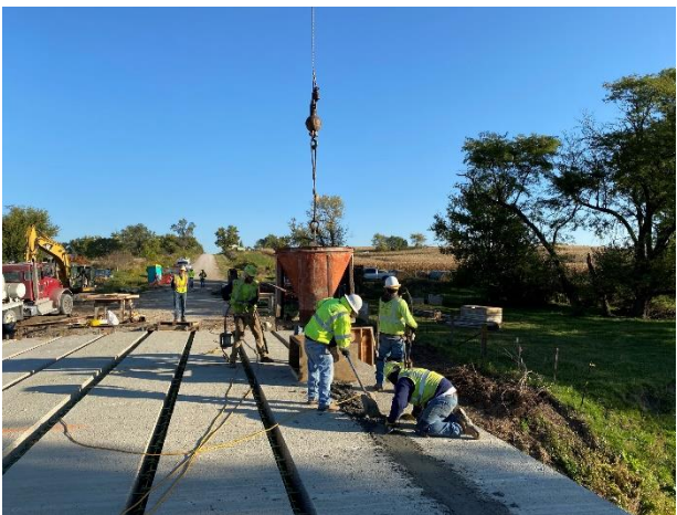
(c) Lifting equipment to move bucket
