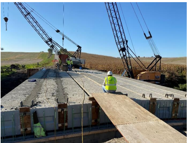
(a) Placement of joint concrete
