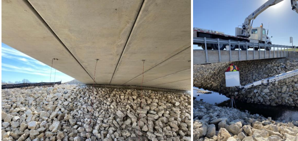
Figure 25. Live load test instrumentation placement
