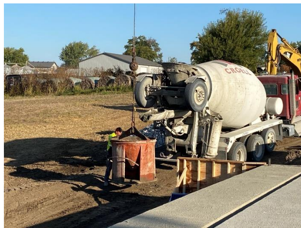
(b) Concrete transfer from truck to bucket
