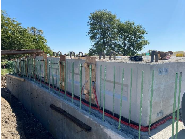
(c) Plywood forms at the ends of the joints
