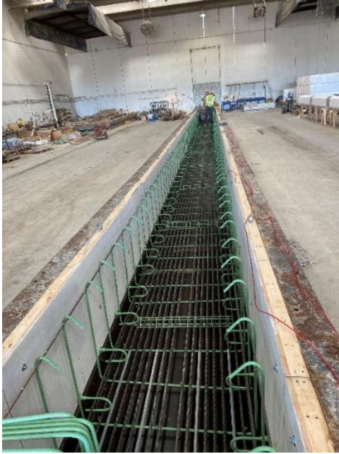
(a) Box girder reinforcement placement
