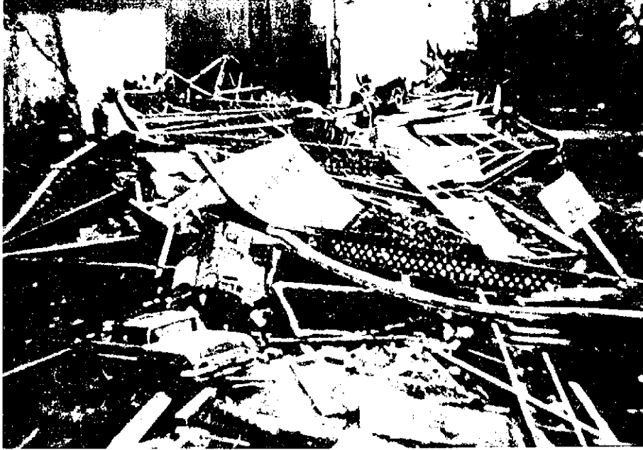
I-2. Pt. Pleasant Bridge after Brittle Fracture
