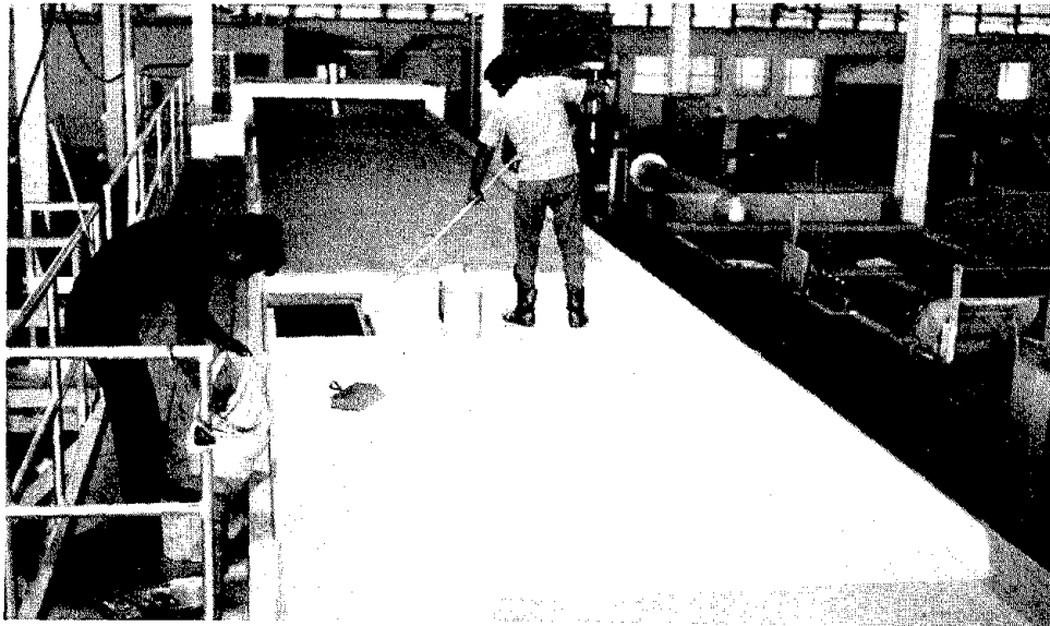
Figure 5-5. - Roadbed surface treatment. Photo H-1765-18
