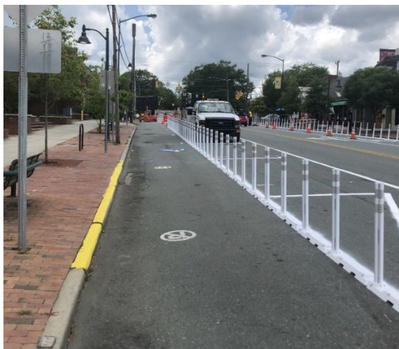
Figure 14. Temporary multiuse path on Franklin St., Chapel Hill, NC. (Image Credit: Town of Chapel Hill)
