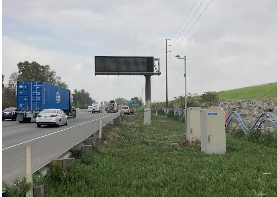
Figure 2-5 Equipment Setup at I-710 Willow
