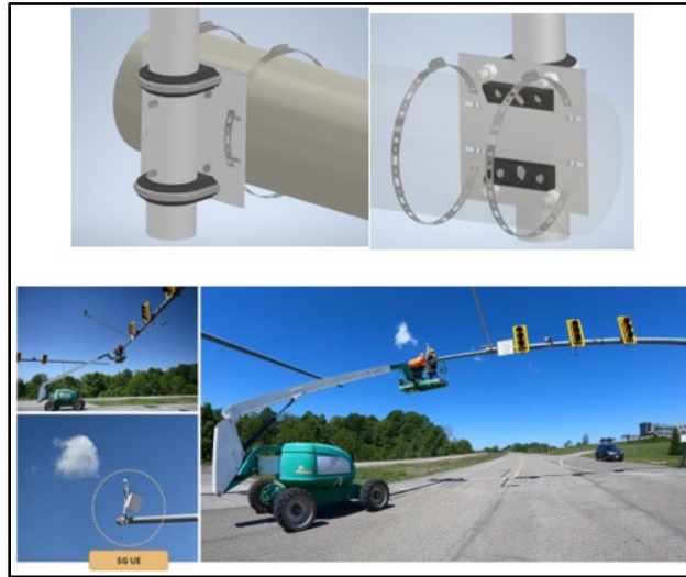
Figure 7. Photos and illustrations. RU mount and installation.
