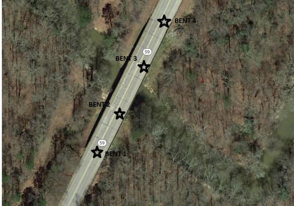
Figure 14. Photo. Overview of the construction site in Banks County, GA.
