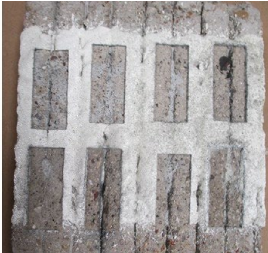
Figure 4: Photograph of a white thermo (by truck) stripe on concrete specimen with different ablated regions.
