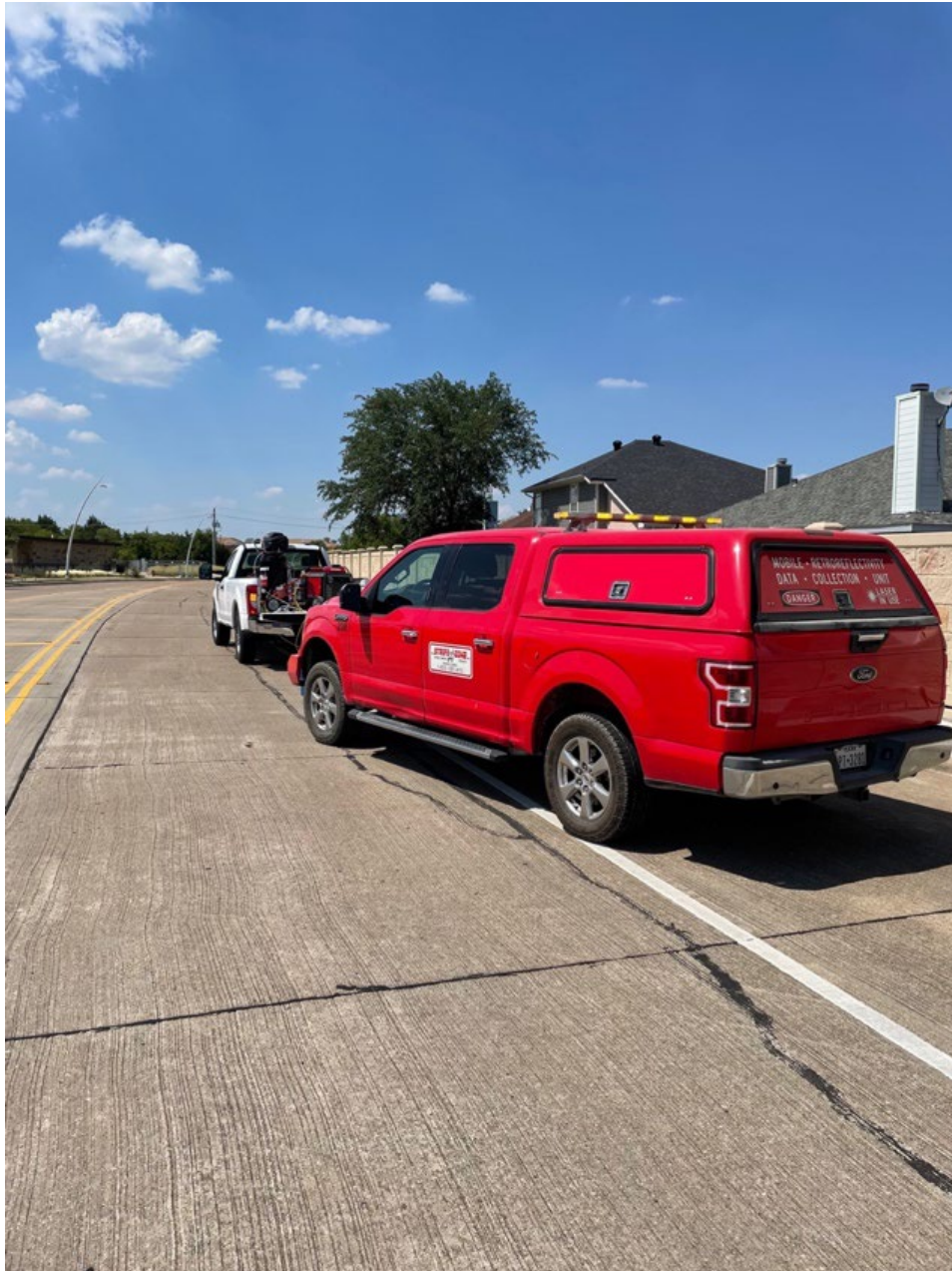
Figure 11: Traffic control during the ablation operations.
