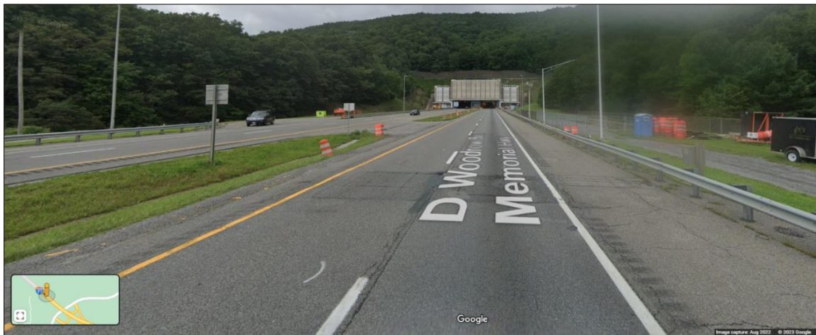
Figure 15. View of the South Entrance of Big Walker Tunnel on I-77 Near the APRS Deployment Site
