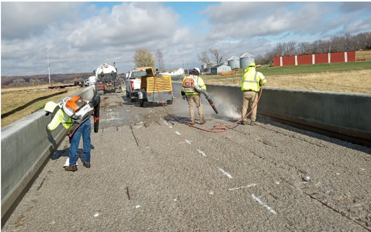
Figure 5.20 Cleaning up of concrete surface after hydrodemolition of Route M Bridge
