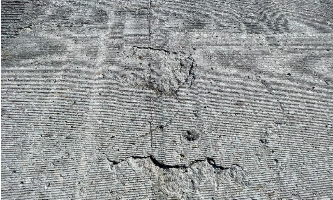
Figure 5.19 (continued) (a) Overview of diamond ground surface for Route Z Bridge (b) close-up view, and (c) cracking of subbase of Route Z Bridge
