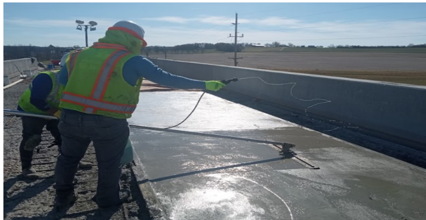
Figure 5.30 Application of evaporation retardant at conclusion of finishing of UHPC
