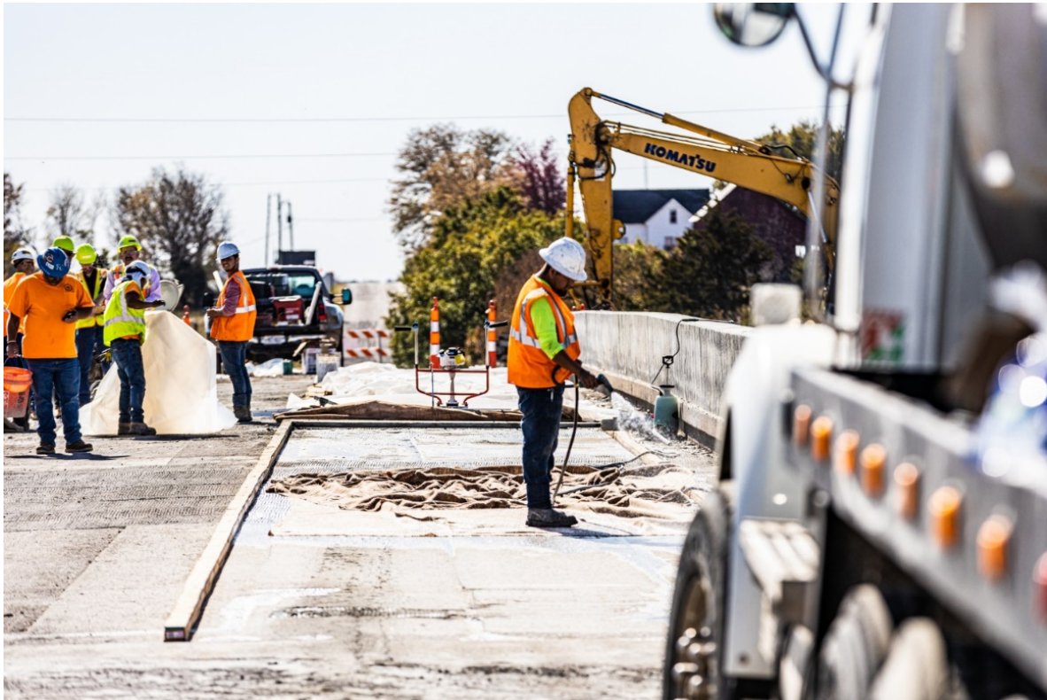
Figure 5.22 Pre-wetting of Route Z Bridge concrete substrate before overlay casting
