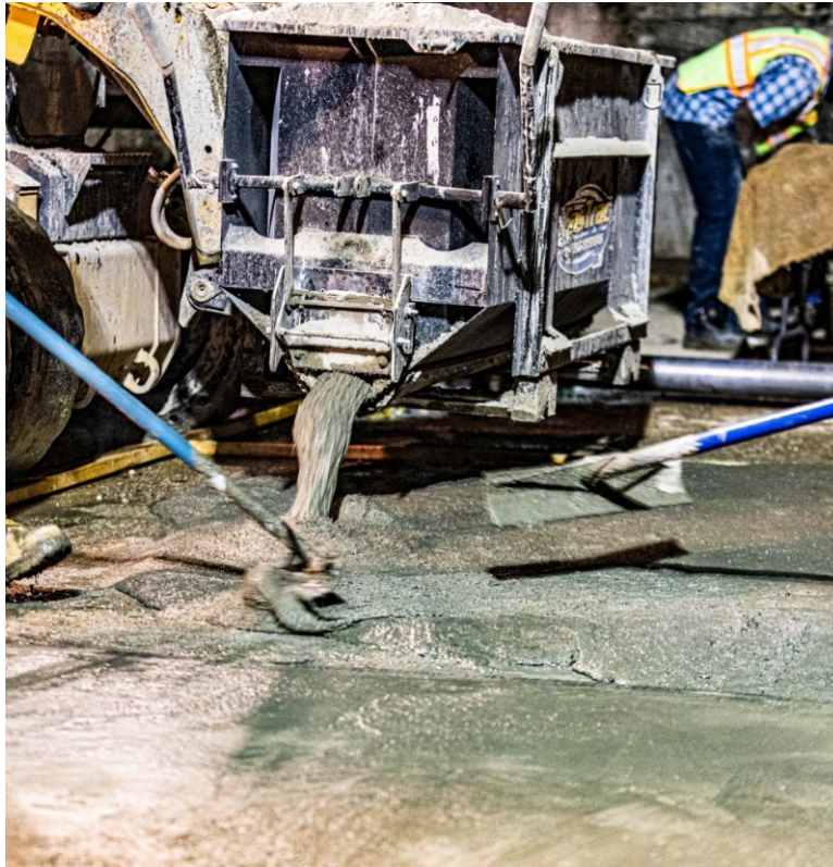
Figure 5.10 Placement of mockup UHPC
