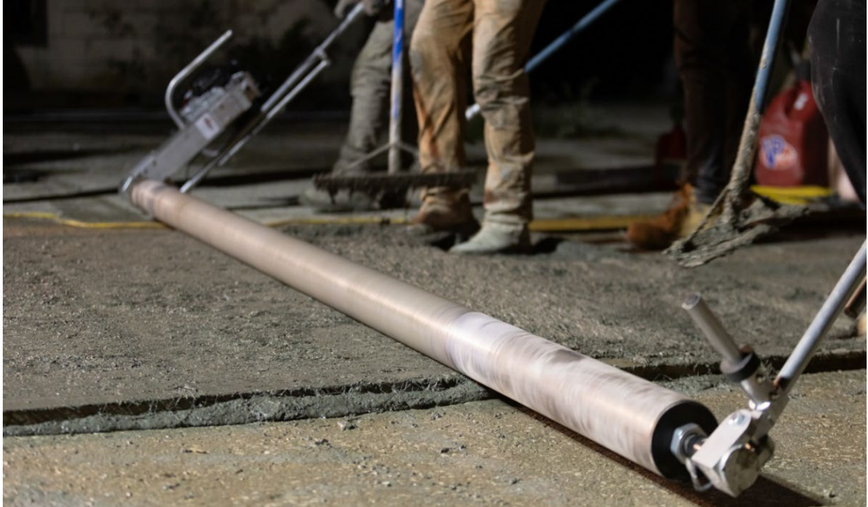
Figure 5.12 Finishing of mockup mixtures with roller screed
