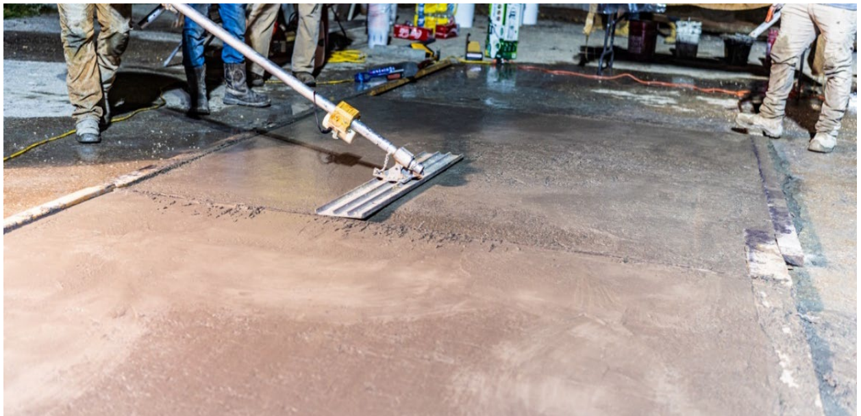
Figure 5.13 Finishing of mockup mixtures with hand-held tools at contractors' property
