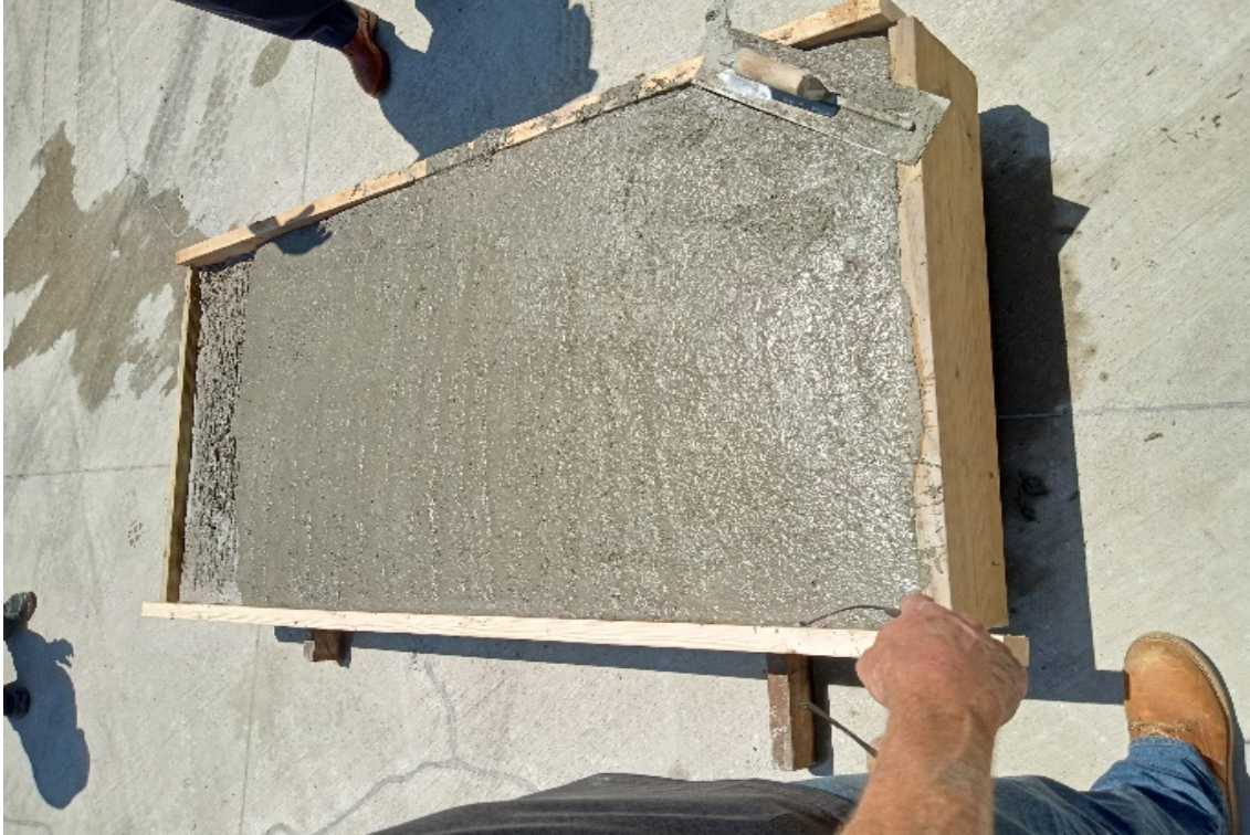
Figure 5.5 Placement of UHPC overlay
