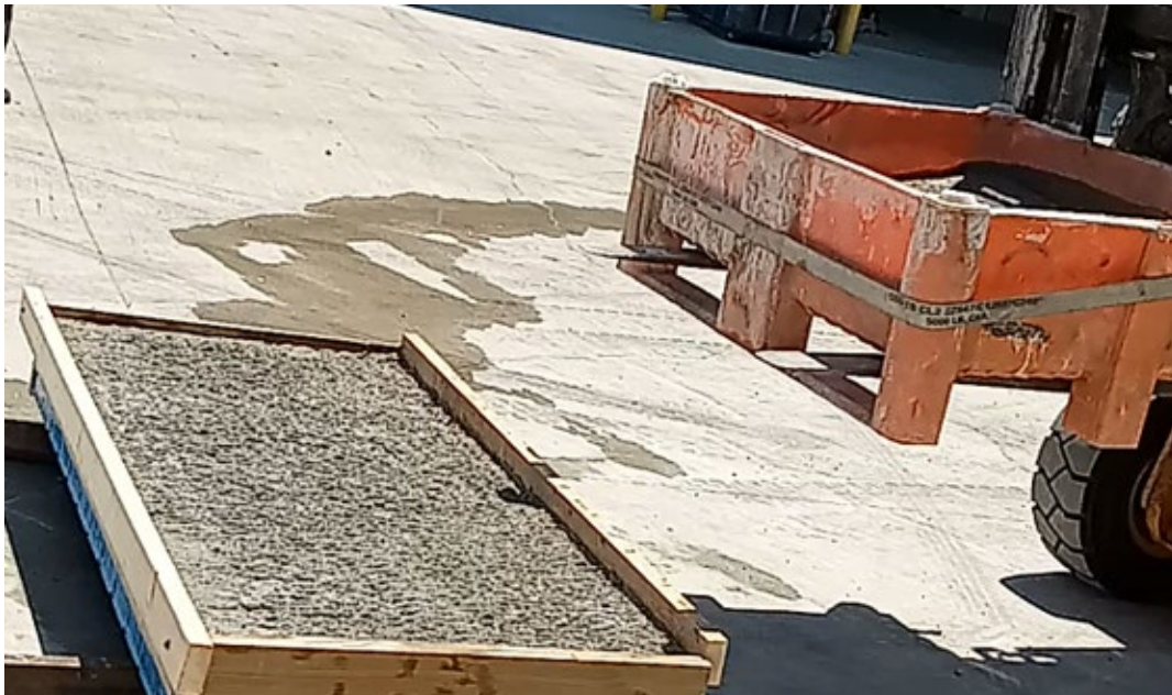
Figure 5.4 UHPC transport onto conventional concrete substrate using forklift
