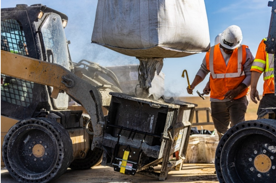
Figure 5.28 Loading of materials into mixer and UHPC mixing
