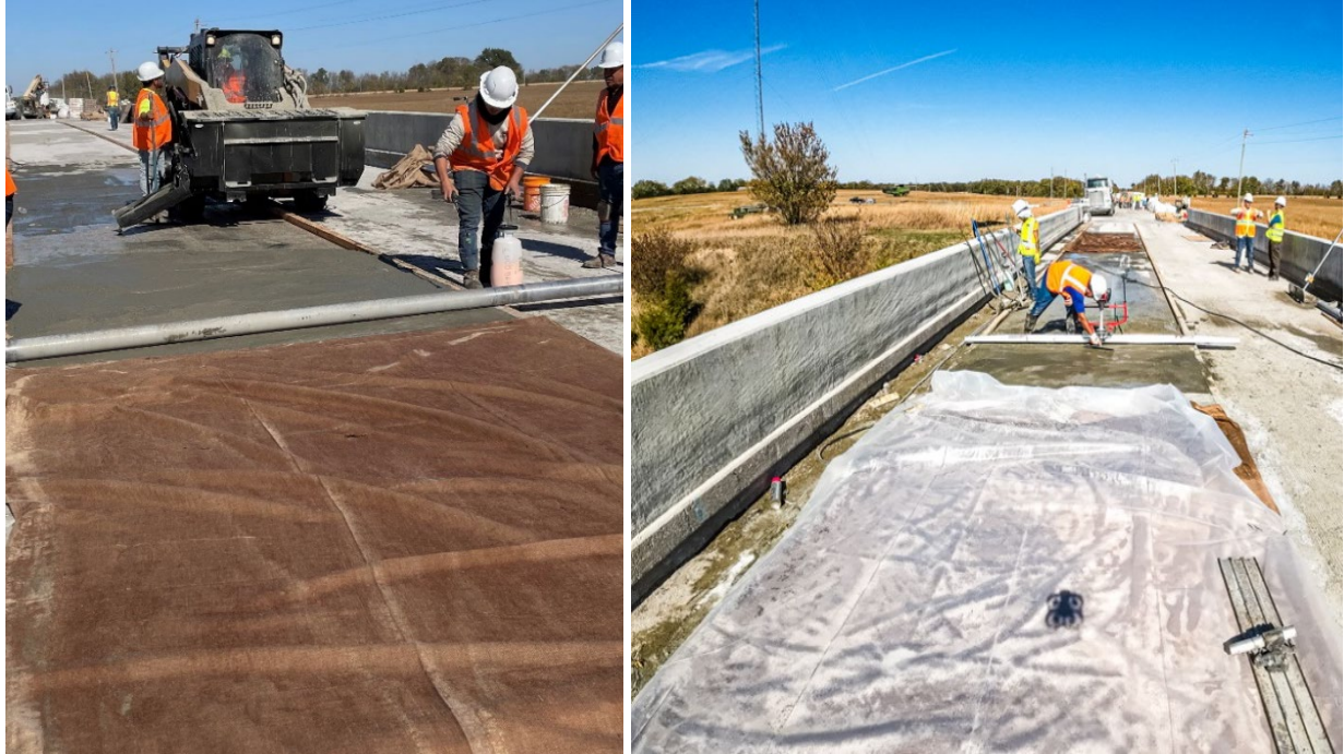
Figure 5.31 Curing of UHPC with evaporation retardant, wet burlap, and plastic sheet
