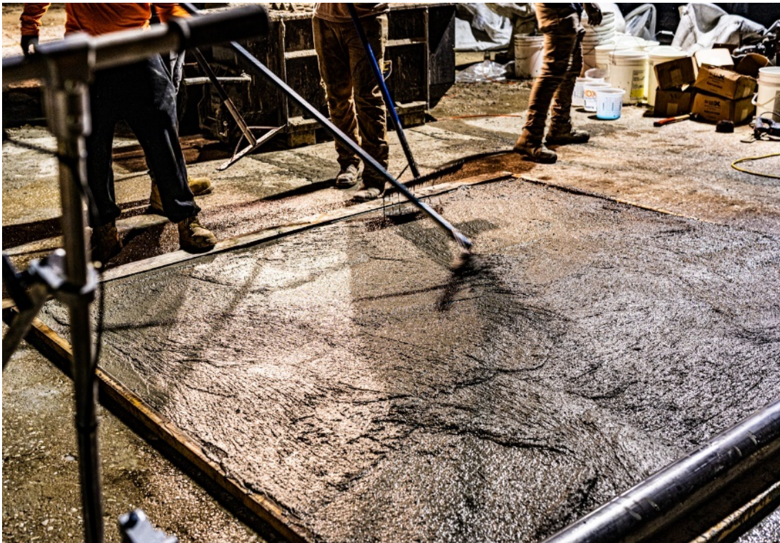
Figure 5.10 Placement of mockup UHPC
