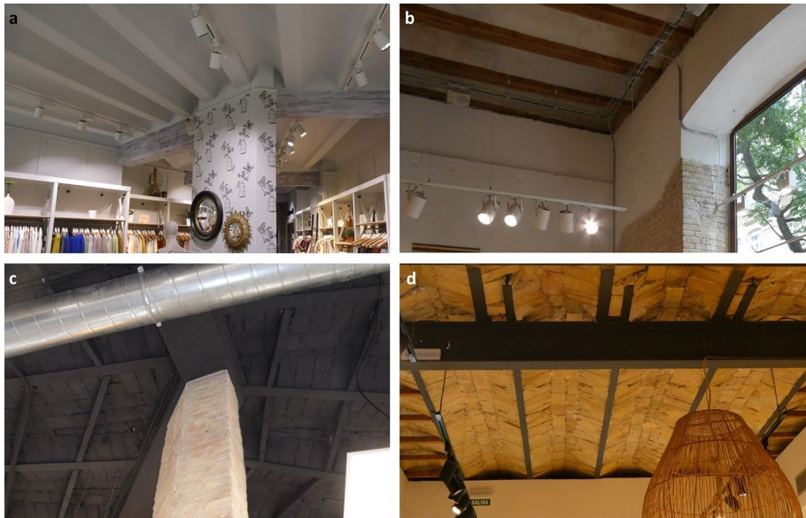
Fig. 14 Structural typologies: a timber beams and joists, b brick masonry bearing wall and timber joists, c brick masonry column with steel beams and joist and d steel beams and light tiles vaults. (Source: Authors 2021–2022)
