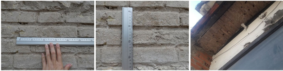
Fig. 16 Dimensions of the brick units and thickness of the façade. (Source: Authors 2022)
