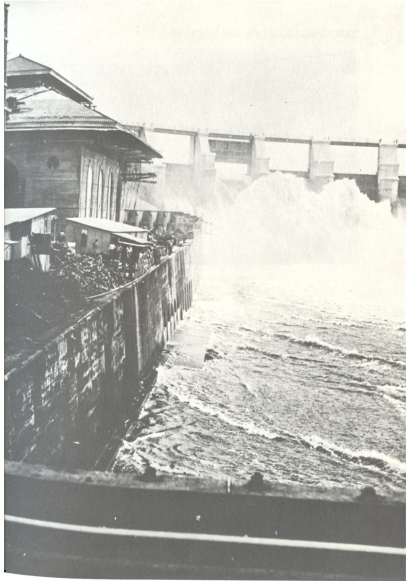
Left and above: Filling Gatun locks for the first time. The building in the upper left corner is the control house from which all the machines on the locks were controlled
