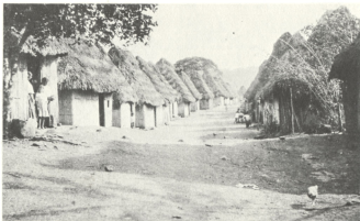
A typical native street of interior of Panama
