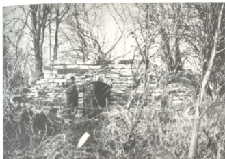
The exterior and grounds of the Fairchild Wine Vault before restoration
