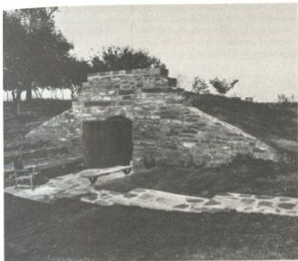
The exterior and grounds of the Fairchild Wine Vault following restoration
