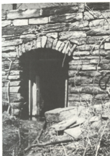
The entrance to the Fairchild Wine Vault before restoration
