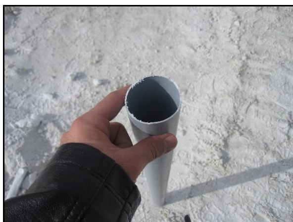
Figure 9. PVC pipe used to create an air deck.
