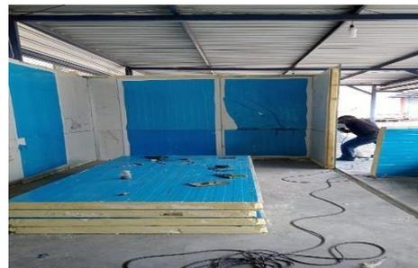
**Gambar 3.** Pemasangan dinding coldstorage
