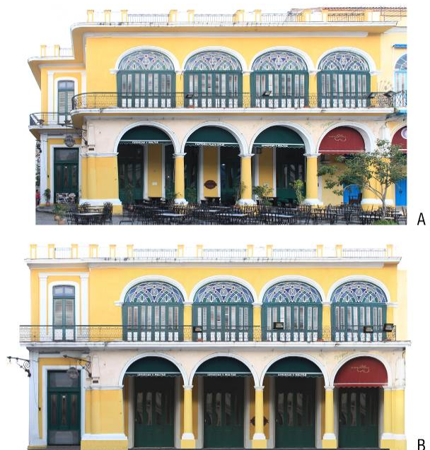
Figure 9. Comparison of the photo rectification (A) and the orthophoto map (B) of a building in Plaza Vieja
