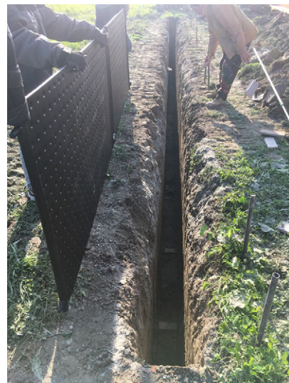
Figure 4. Flat-Panels and trench.
