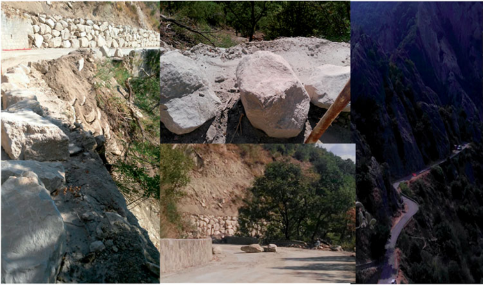
Figure 12. Mass movement event occurred in “Margiass” location (14 April 2017).
