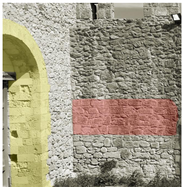
Figure 3. The medieval courtyard of the castle of Mussomeli with different materials used on different stages of restoration (in red and in yellow).
