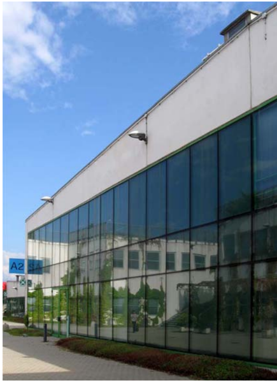
FIGURE 4. The Climate Façade tested in-situ.
