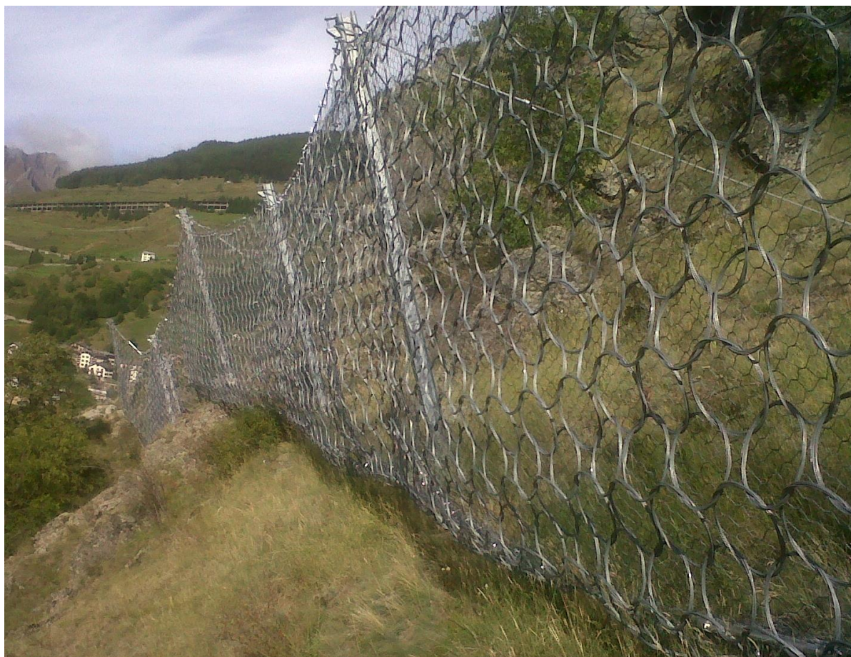
Figure 1 - Photo of the rockfall protection net fence studied
