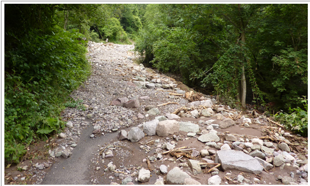
Figure 9 - A forest road classified as virtual reach affected by runoff triggered by an intense storm.
