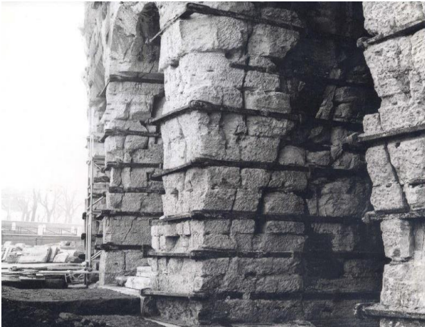
Figure 4. Image related to the retrofit interventions carried out in the 1970, that shows the state of the columns.
