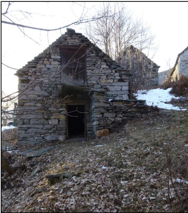
Figure 2. Typical Alpine stone building
