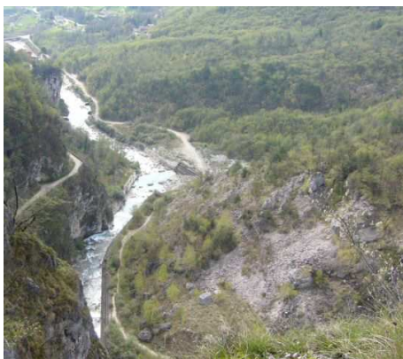
Figure 2: View of the bottom side of the landslide.
