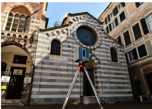
Figure 7. Scan position to acquire the point cloud of the Chiesa di S. Matteo facade (R. Lavezzaro)
