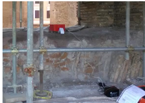
Figure 4. Instrumentation setup: position C.
