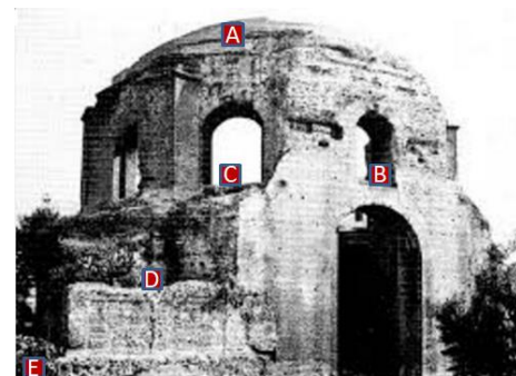
Figure 2. Measurement points on the main façade (view from North).
