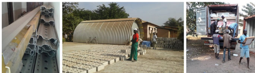
Fig. 9 Materials selection, transportation, and preparation for the construction site
