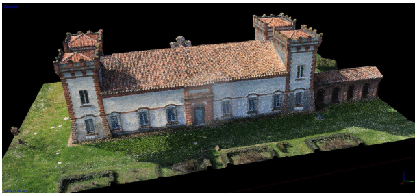
Figure 19. Back view of the final model.
