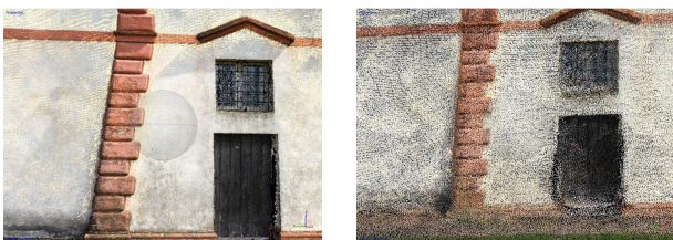
Figure 20. The images above show the difference between the point cloud of model M3 (on the left) and the one obtained from the unique model (on the right). The comparison shows the higher definition of the first one.
