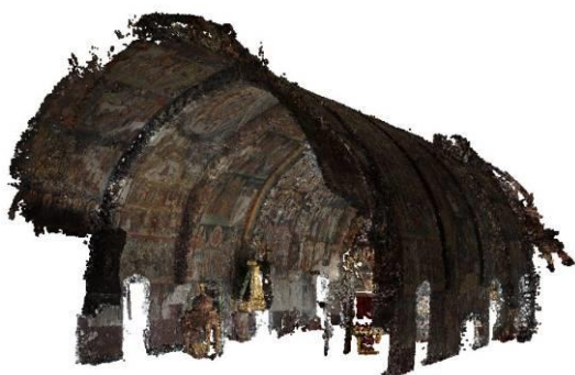
Figure 9. Dense cloud reconstruction of the barrel vault
