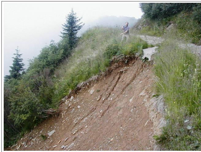
Figure 1 - Example of road induced landslide on the Eastern Italian Alps [picture courtesy of Cazorzi F.].
