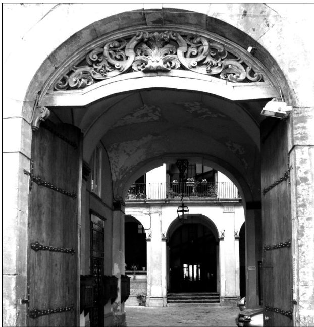
Fig.7. Entrance to the Main Courtyard
