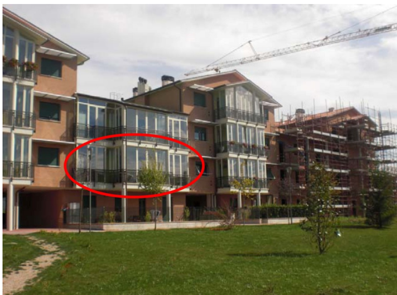
Figure 5. View of the south-west façade of the building, with the flat used as case study.
