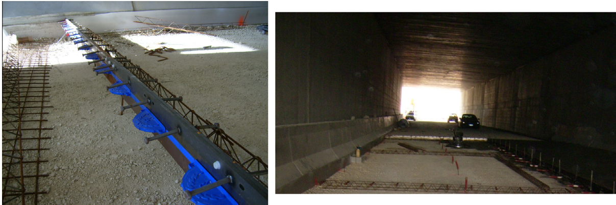
Fig. 3. Transverse (left) and longitudinal (right) joints.
