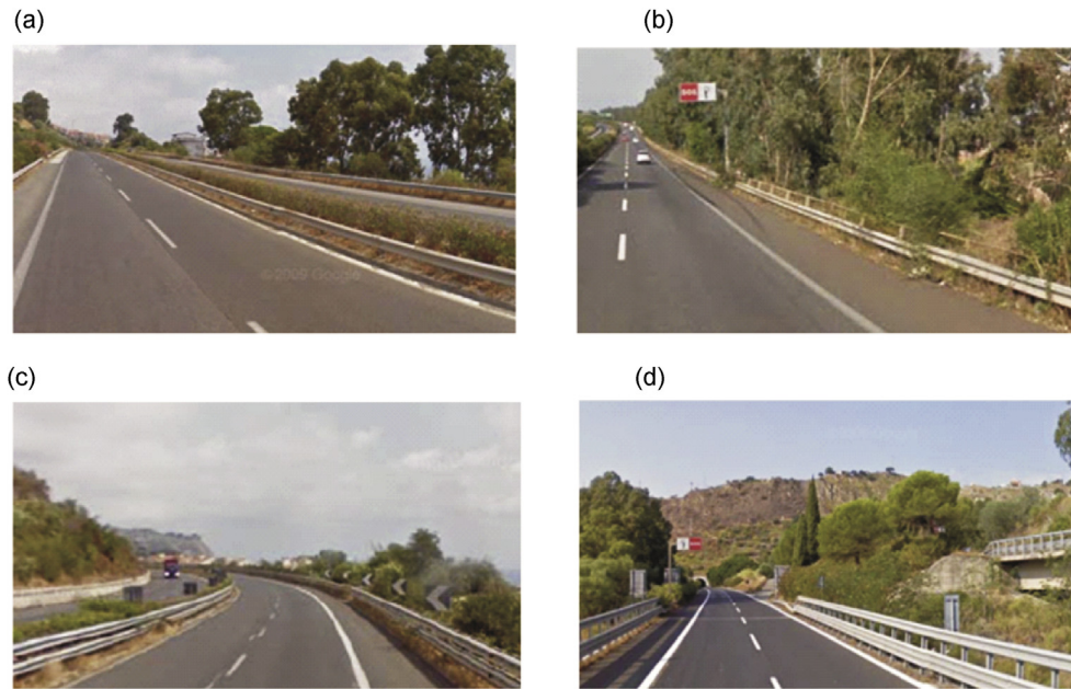
Fig. 1 – Pictures of barriers installed on a motorway in Italy. (a) Old barriers on the embankment. (b) Old barriers on the bridge. (c) New barriers on the embankment. (d) New barriers on the bridge.
