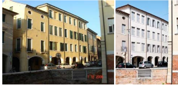
Fig. 1 General view of the building a) before and b) after the intervention.
