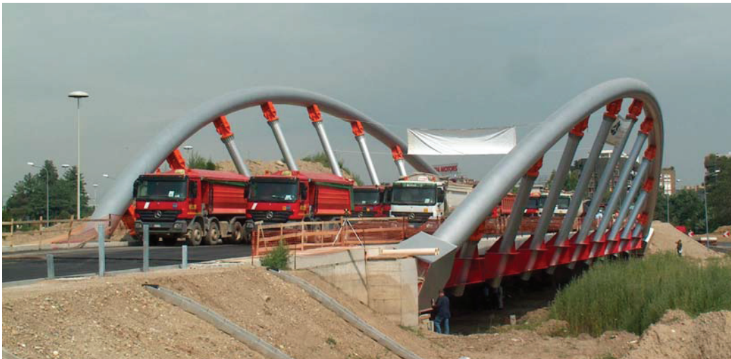
Figure 1: The De Gasperi Bridge during loading test.
