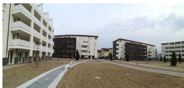
Fig. 5. Photos of the new social housing residences
