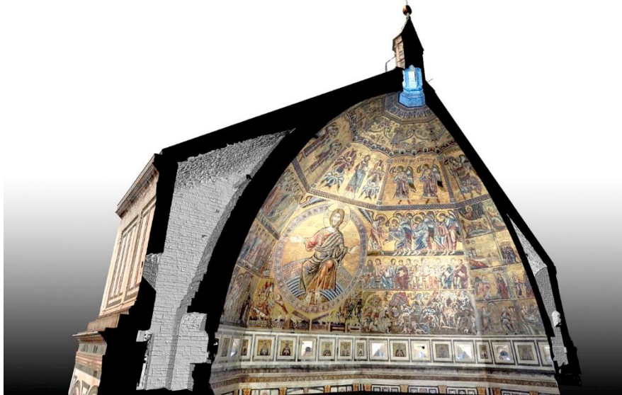
Fig. 2. Florence Baptistery: 3D model with a detail of the extrados of the dome.
