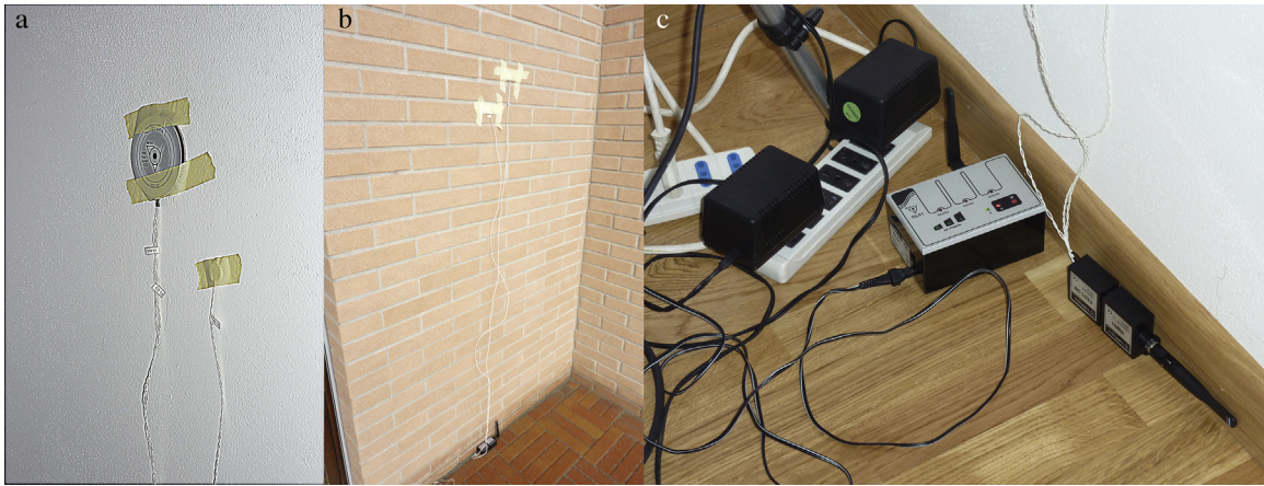
Fig. 3. Installation of the sensors on a tested wall: (a) inner surface of the wall; (b) outer surface of the wall; (c) acquisition system.
