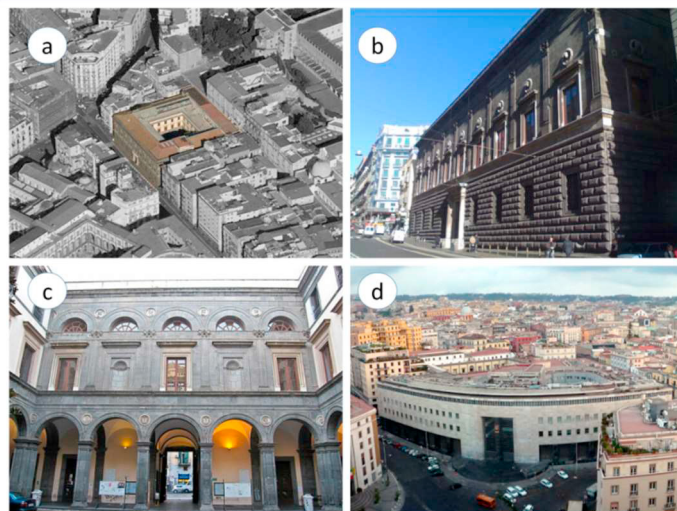
Fig. 1. Palazzo Gravina: overview (a), main façade (b), courtyard (c), near post-office (d)
